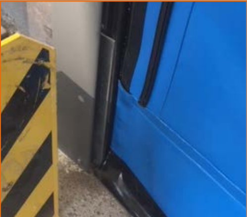
Guide rail with zip system and FlexEdge bottom bar
