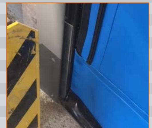
Guide rail with zip system and FlexEdge bottom bar
